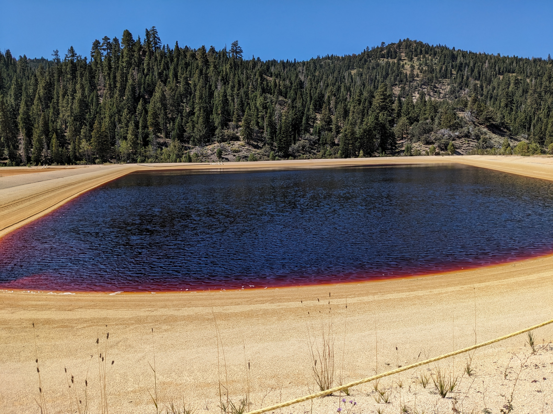
Pond 2 South: part of the pond water treatment system
