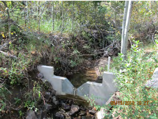
New weir located on 4L Creek
