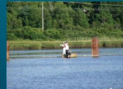
Steel cables that span the sheet piles
