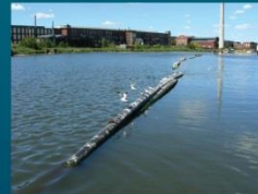
Floating and submerged pipelines
